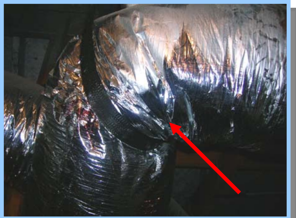
SHARP DUCT BENDS REDUCE AIR FLOW
