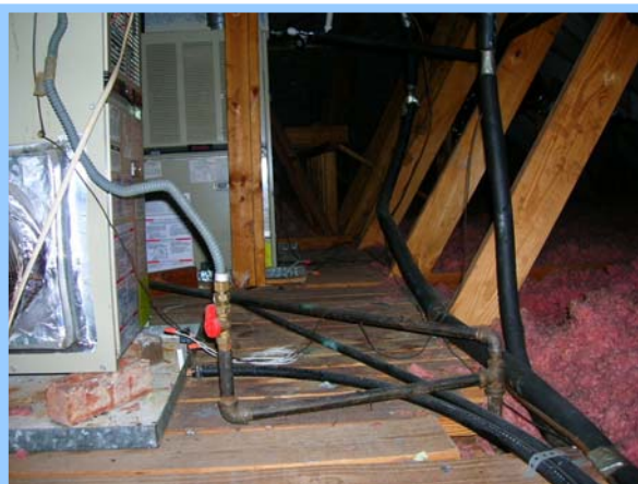
PIPING ON ATTIC FLOOR RESTRICTS ACCESS TO VARIOUS MECHANICAL EQUIPMENT
