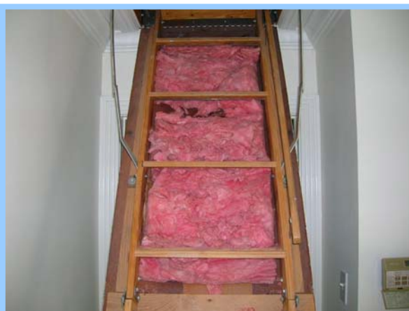
REMOVE INSULATION BATTS ON STAIRWAY
