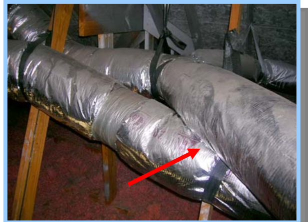
DUCTS SHOULD NOT TOUCH OTHER DUCTS
