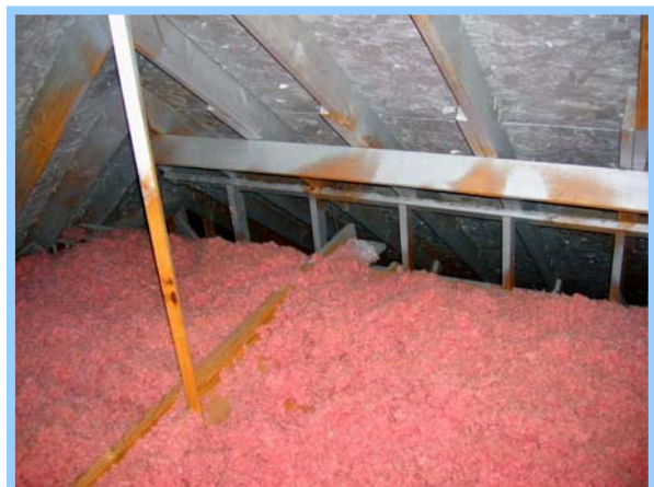
LOOSE FILL FIBERGLASS INSULATION
